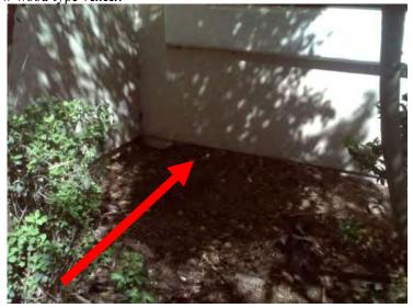
The soil line at the south west corner is marginally high. Under current building standards there should be at least 4-inches of foundation visible below masonry veneer and 6-inches of foundation visible below wood type veneer.
