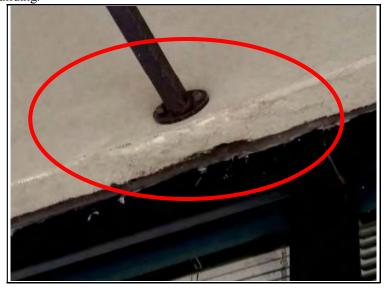
One or more locations at the parapet wall transitions need to be re-sealed.
