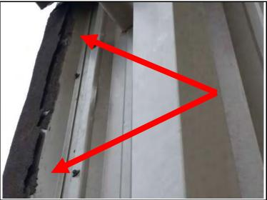
NOTE: Previous repairs to the stucco veneer (EIFS) were observed at a few locations along the front of the building.
