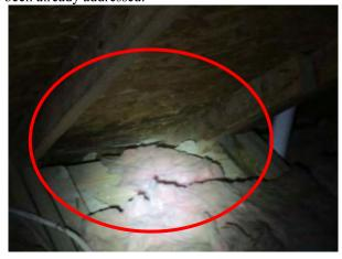
The ridge board should be the full depth of the cut rafters. This is a common observation in older homes and may have not been required at the time your house was built, although per TREC standards I am required to report this item as in need of repair.
