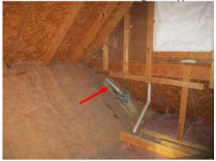
Loose fitting joints and/or openings in the ductwork should be improved at many locations.
