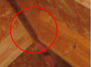
There is a damage truss gusset connection in the east area of the upper attic. This area should be investigated and/or repaired.
