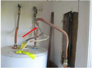
Some corrosion was observed at the water supply connections at the top of the water heater.
