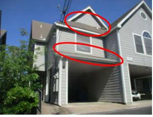
There was no kickout flashing details observed at the lower bottom edge of the roof line interface and the sidewall that continues past the edge of the roof. The lack of this kickout flashing can allow water to penetrate at these points.
