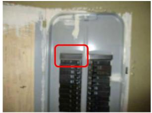
Double wired/lugged neutral wires observed in the sub panel. The arrangement is considered improper.
