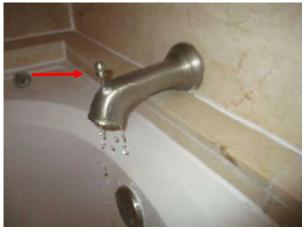
The supply valves and faucet for the shower/tub should be sealed to the enclosure.
