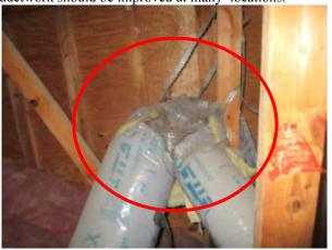
The ducts are leaking air where they attach to the supply plenum. This should be repaired to improve efficiency.
