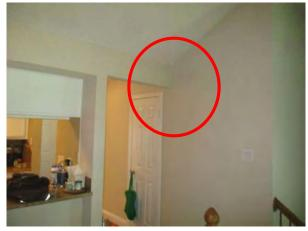
Wall sheetrock stress cracks were observed in upstairs kitchen hall.
