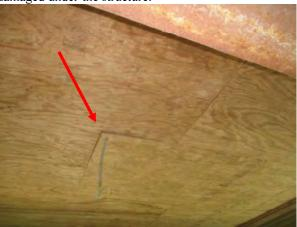
Water stains were observed on the ceiling finish material under the structure. The cause and remedy should be further evaluated and corrected as necessary.
