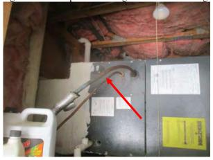
It appears the cover to the evaporator coil is not sealed and is drawing air from within the attic space. Recommend repair by a licensed HVAC technician.
