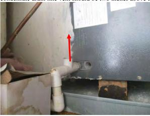
Damaged, deteriorated and/or missing insulation on the refrigerant lines at the evaporator coil should be repaired or replaced as necessary. This will keep condensate from dripping into the pan and potentially causing corrosion and possible damage to floors and ceilings.
