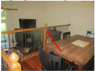
One of the stair balusters is missing and should be replaced for safety reasons.
