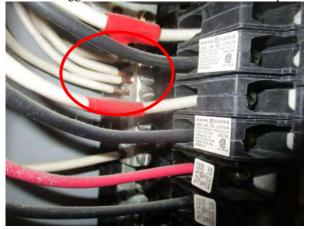
One or more of the breaker trip-ties appear to be missing. The 120V overcurrent devices (breakers) sharing a grounded conductor (Neutral) should be connected together by trip-ties. This is a common observation for a home of this age and under TREC standards of practice I must list this item as deficient.
