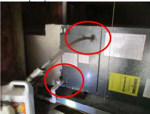
There is air leaking where the supply air plenum attaches to the air handler. This improvement is a minor repair and will reduce energy costs.
