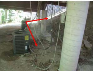
The primary condensate drain lines are not equipped with a p-trap. Under current mechanical installation standards, the manufacturer requires a p-trap be installed in the primary condensate drain line within 6-inches of the coil housing.
