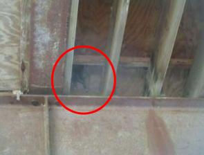
No safety pan and drain was found for the water heater. This should be repaired by the installation of a pan with a drain by a qualified professional
