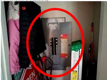
One or more of the breaker trip-ties appear to be missing. The 120V overcurrent devices (breakers) sharing a grounded conductor (Neutral) should be connected together by trip-ties.
