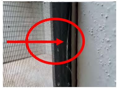
The window(s) adjacent the front door was observed to be broken or cracked.
