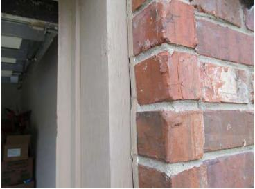
Gaps in the exterior veneer should be sealed in various locations to prevent water infiltration. This is an aspect of regular home maintenance.
